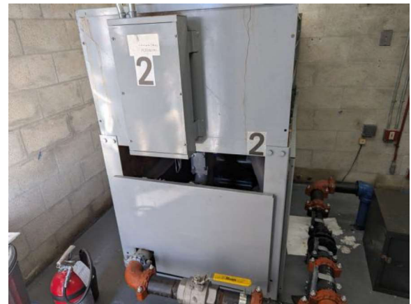
LKMC017e 1/27/2026 Hydraulic plant for passenger elevator ELEV-2 Elevator mechanical penthouse
