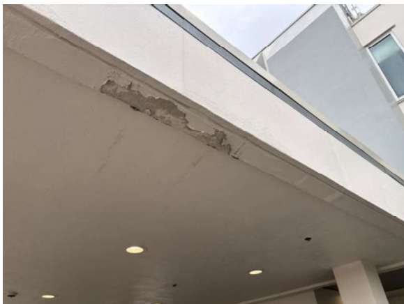
LKMC116a 1/27/2026 Compromised painted stucco exterior ceiling North entry canopy
