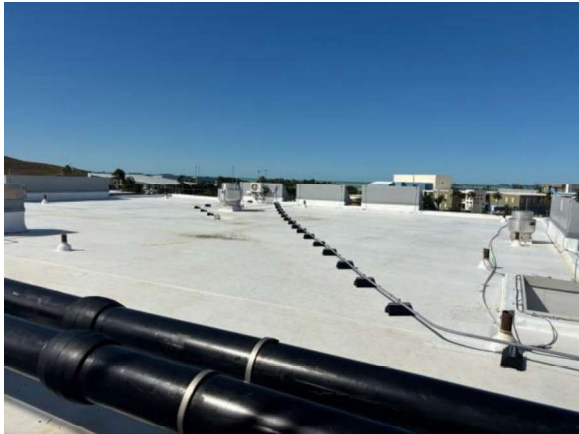
LKMC007a 1/27/2026 Flat single-ply white membrane roof lacking tie-offs Upper roof
