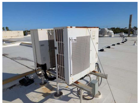
LKMC029e 1/27/2026 Air-cooled condenser for ductless split systems DDXS-4 and DDXS-5 East lower roof
