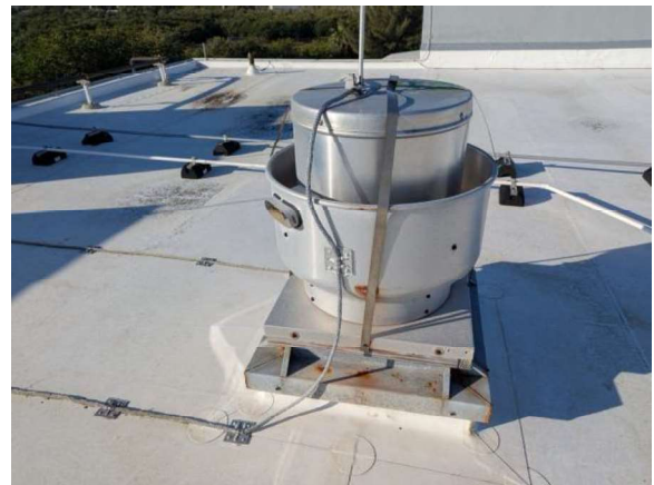
LKMC011e 1/27/2026 Centrifugal curb-mounted exhauster 3-3 Upper roof
