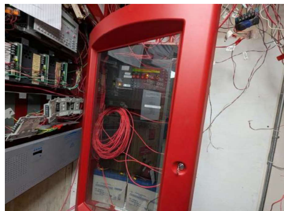
LKMC108e 1/27/2026 Simplex 4100ES fire alarm control panel FA/COMM room
