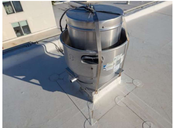
LKMC004e 1/27/2026 Centrifugal curb-mounted exhauster EF-ICU Upper roof
