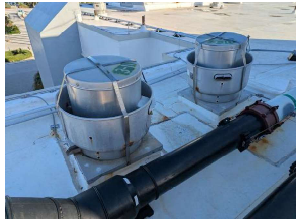
LKMC007e 1/27/2026 Centrifugal curb-mounted exhausters 3-10 and 3-11 Upper roof
