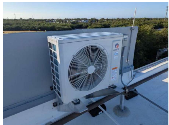
LKMC012e 1/27/2026 Air-cooled condenser for ductless split system DDXS-B Upper roof
