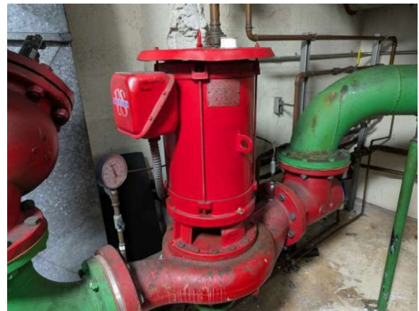
LKMC077e 1/27/2026 Condenser water pump CW-2 Chiller room
