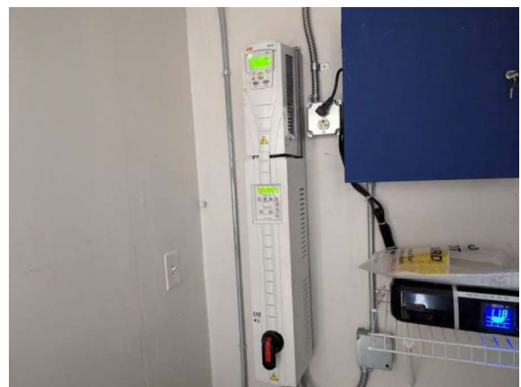
Variable frequency drive AHU-12 VFD Second floor, northwest mechanical room
