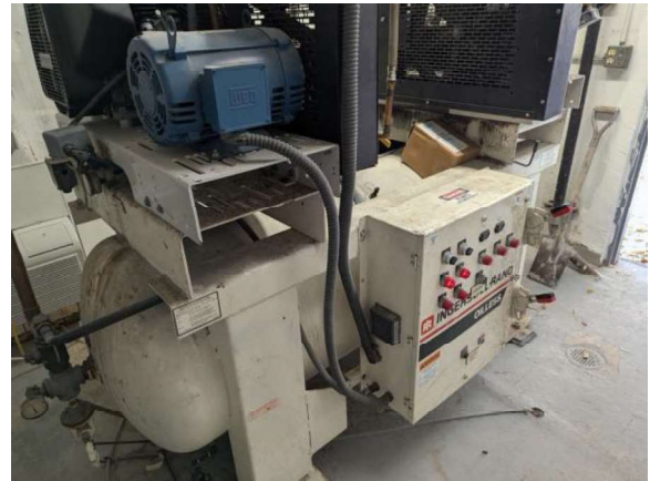
LKMC061e 1/27/2026 Duplex medical air compressor MAC-1 Compressor room
