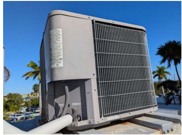
LKMC046e 1/27/2026 Ducted split system air-cooled condenser 3 North lower roof
