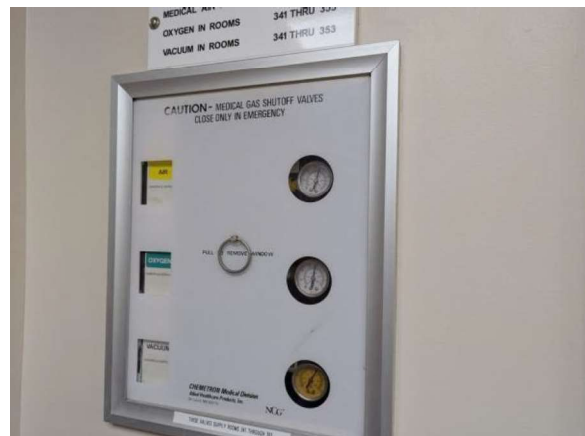
LKMC117e 1/27/2026 Analog medical gas panel Suite 3-D
