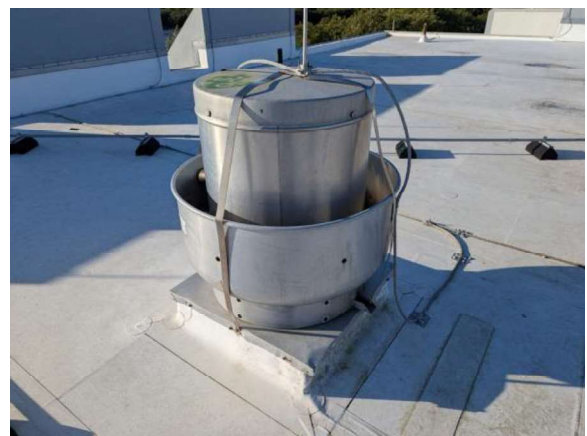
LKMC002e 1/27/2026 Centrifugal curb-mounted exhauster 3-6 Upper roof
