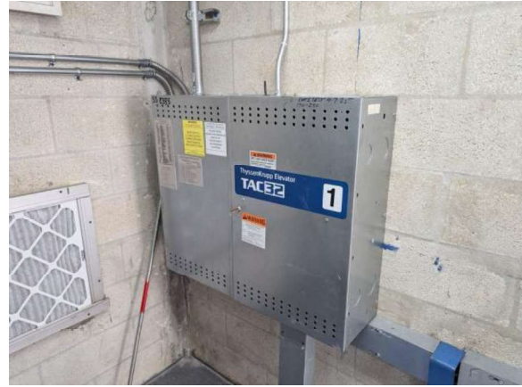
LKMC019e 1/27/2026 Solid state control panel for passenger elevator, ELEV-2 Elevator mechanical penthouse
