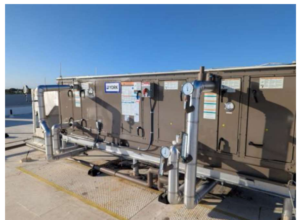
LKMC003e 1/27/2026 Outdoor air handler RTU-3A Upper roof
