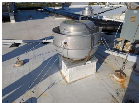
LKMC006e 1/27/2026 Centrifugal curb-mounted exhauster EF-2 Upper roof
