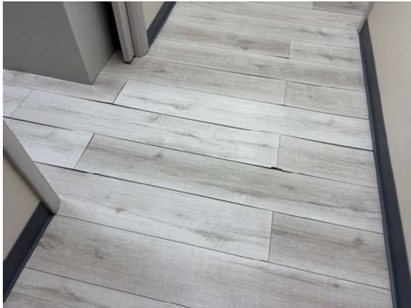
LKMC100a 1/27/2026 Compromised vinyl plank First floor, Business building corridor
