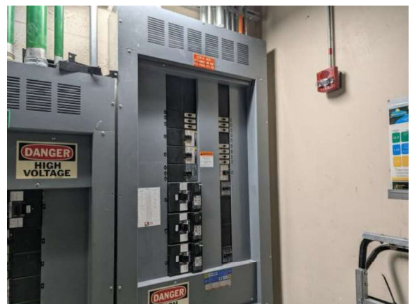
LKMC101e 1/27/2026 Electrical distribution load center CDP/A Electrical room
