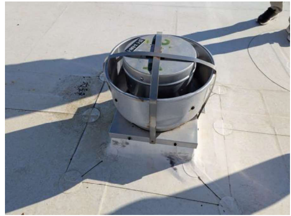
LKMC028e 1/27/2026 Centrifugal curb-mounted exhauster EF-1 X-RAY-1 East lower roof
