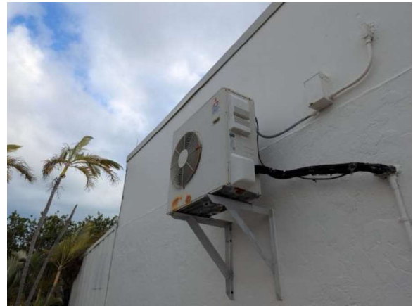
LKMC147e 1/27/2026 Air-cooled condenser for ductless split system DDXS-1 East elevation
