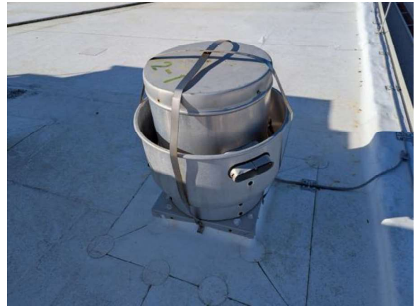
LKMC037e 1/27/2026 Centrifugal curb-mounted exhauster 2-1 East lower roof
