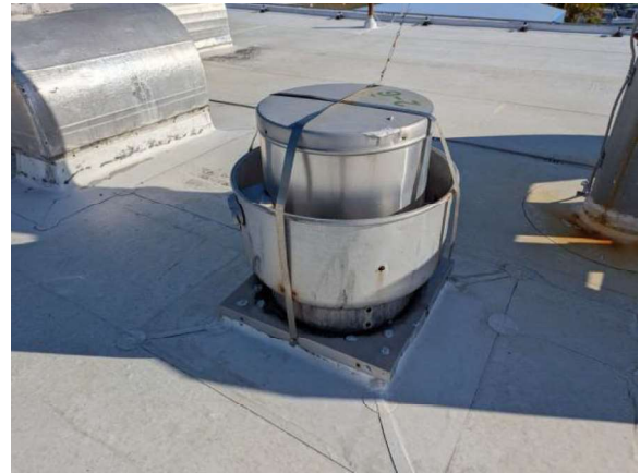
LKMC031e 1/27/2026 Centrifugal curb-mounted exhauster 2-6 East lower roof
