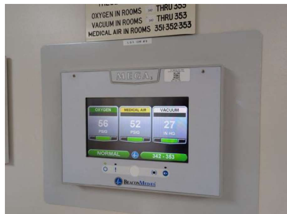
LKMC116e 1/27/2026 Digital medical gas panel Suite 3-D
