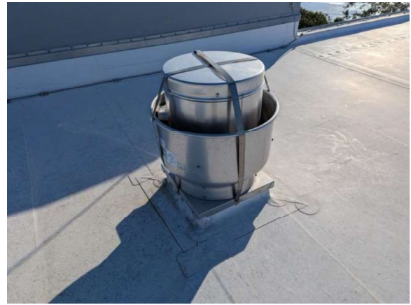
LKMC010e 1/27/2026 Centrifugal curb-mounted exhauster EF-3-4 Upper roof
