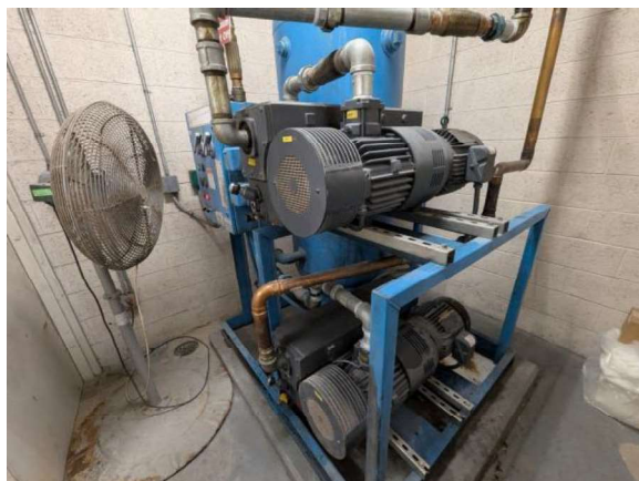
LKMC124e 1/27/2026 Duplex vacuum pump VACP-2 Medical vacuum pump room
