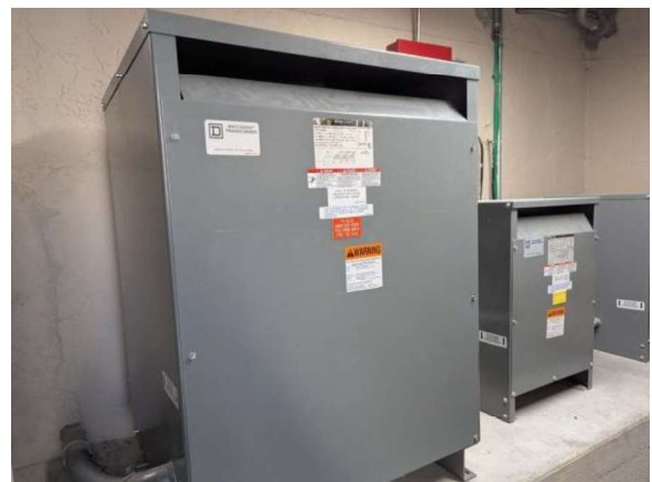
LKMC105e 1/27/2026 Electrical distribution transformer, TX-1C/A Electrical room
