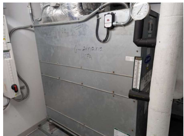
Indoor air handler AHU-12A Second floor, west mechanical room
