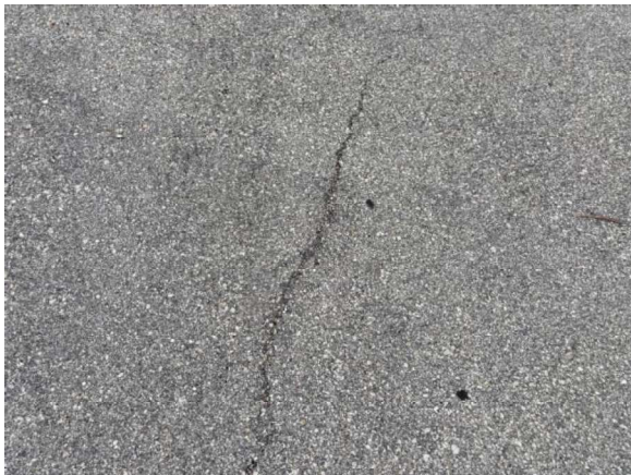
LKMC119a 1/27/2026 Cracked asphaltic concrete North side
