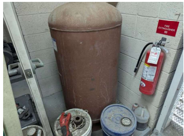
LKMC123e 1/27/2026 Domestic water expansion tank First floor, southwest equipment room
