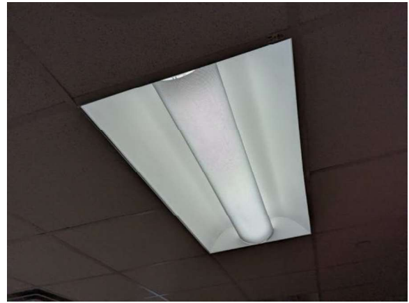
LKMC118e 1/27/2026 Lay-in fixture with T8 fluorescent lamps and acrylic lens Suite 2-C
