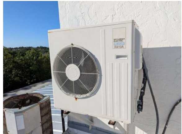
LKMC025e 1/27/2026 Air-cooled condenser for ductless split system DDXS-3 East lower roof
