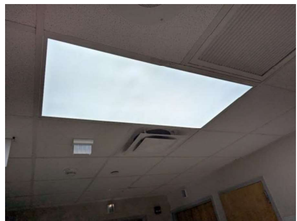
LKMC110e 1/27/2026 Lay-in LED fixture Suite 3-D
