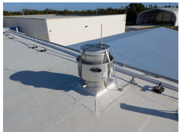
LKMC033e 1/27/2026 Centrifugal curb-mounted exhauster EF-2-2 East lower roof
