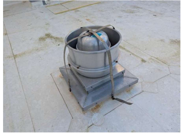
LKMC049e 1/27/2026 Centrifugal curb-mounted exhauster K-5 North lower roof
