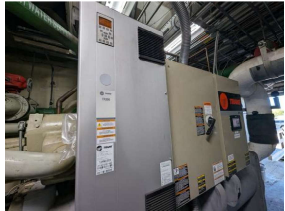
LKMC076e 1/27/2026 Variable frequency drive for chiller 2 Chiller room
