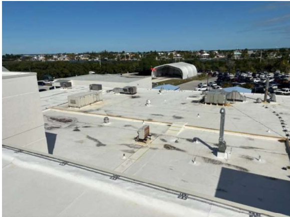
LKMC004a 1/27/2026 Flat single-ply white membrane roof lacking tie-offs Lower roof
