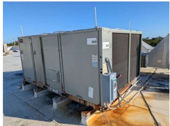
LKMC032e 1/27/2026 Package air conditioning unit RTU-5 East lower roof
