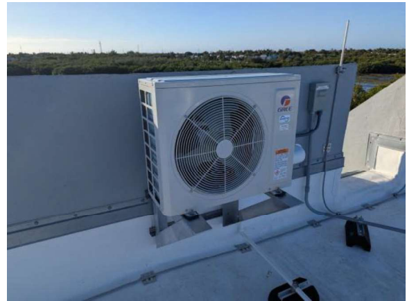
LKMC001e 1/27/2026 Air-cooled condenser for ductless split system DDXS-C Upper roof
