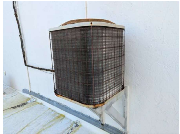
LKMC050e 1/27/2026 Ducted split system air-cooled condenser CNDR-10 North lower roof
