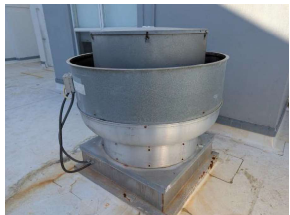
LKMC047e 1/27/2026 Centrifugal curb-mounted exhauster K-2 North lower roof
