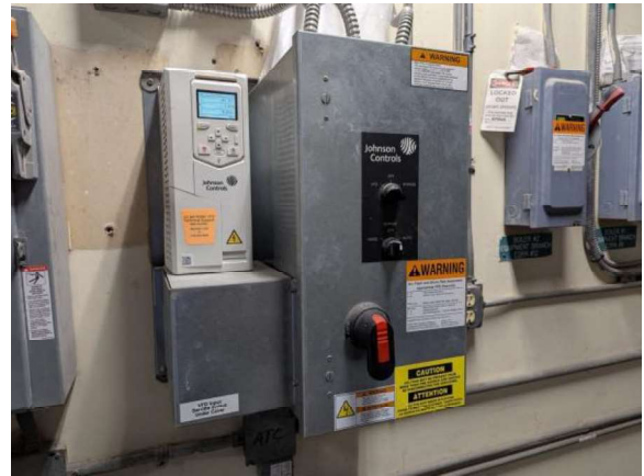
LKMC097e 1/27/2026 Variable frequency drive AHU-21 VFD Boiler room
