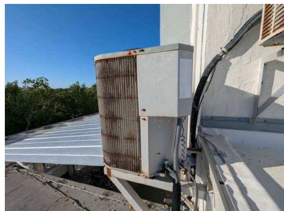
LKMC021e 1/27/2026 Ducted split system air-cooled condenser CNDR-8 East lower roof
