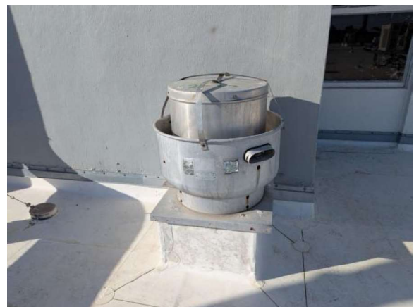
LKMC027e 1/27/2026 Centrifugal curb-mounted exhauster 2-13 East lower roof
