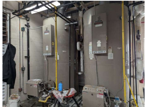
LKMC121e 1/27/2026 Natural gas-fired domestic water boilers 1 and 2 First floor, southwest equipment room
