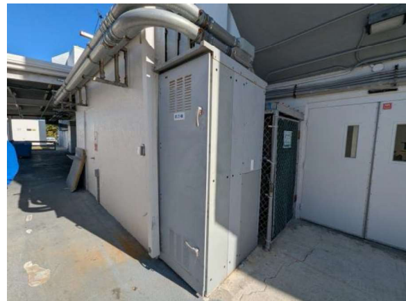
LKMC107e 1/27/2026 Portable generator connection cabinet West elevation
