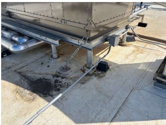
LKMC006a 1/27/2026 Single-ply white membrane penetration detail Upper roof
