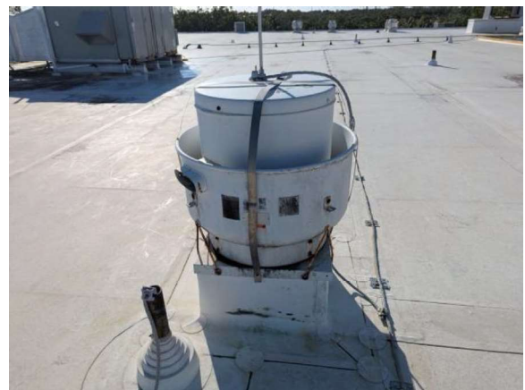
LKMC039e 1/27/2026 Centrifugal curb-mounted exhauster EF1C.1 East lower roof
