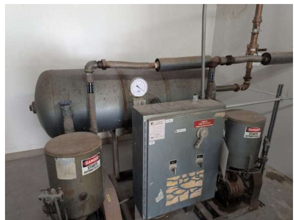
LKMC062e 1/27/2026 Duplex vacuum pump VACP-1 Compressor room
