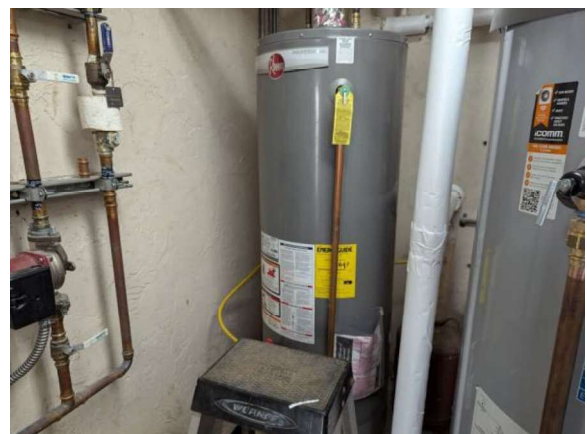
LKMC120e 1/27/2026 Residential-grade, natural gas-fired domestic water heater DHW-3 First floor, southwest equipment room
