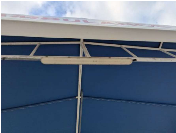
LKMC146e 1/27/2026 Surface-mounted fixture with T8 fluorescent lamps East elevation
