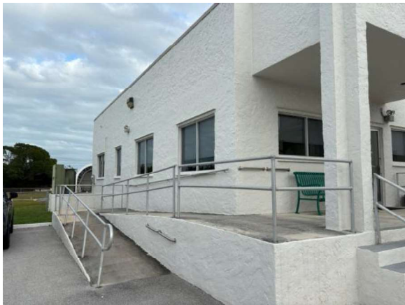
LKMC104a 1/27/2026 Elevated walk with noncompliant guardrail and ramp with noncompliant assemblies Northeast corner
