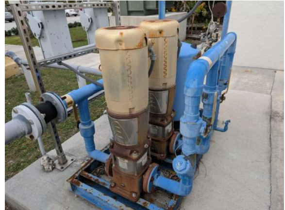
LKMC151e 1/27/2026 Water storage tank transfer pumps 1 and 2 Northwest elevation
