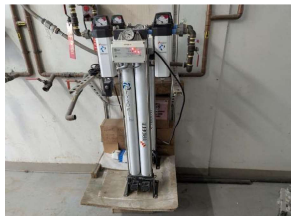
LKMC063e 1/27/2026 Desiccant air dryer for air compressor MAC-1 Compressor room
