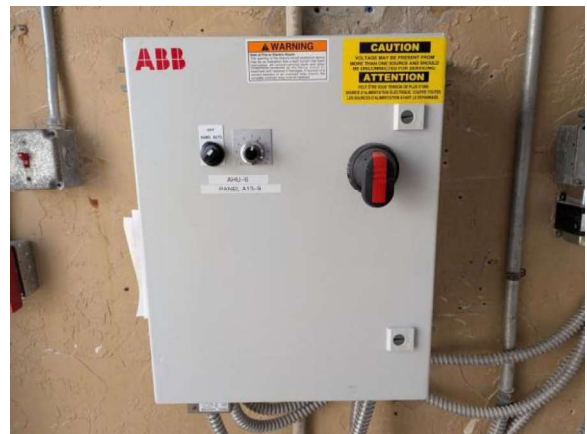
LKMC066e 1/27/2026 Variable frequency drive AHU-6 VFD First floor, southeast mechanical room
