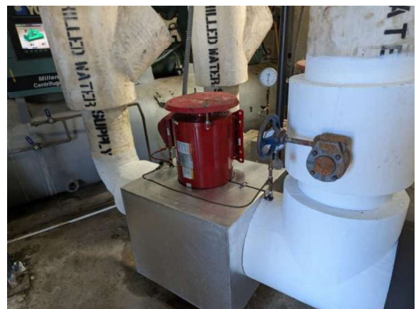
LKMC080e 1/27/2026 Chilled water pump CHW-2 Chiller room
