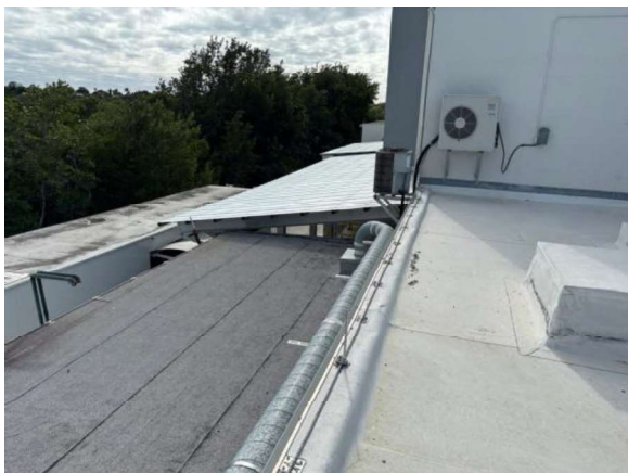
Single-ply membrane, built-up roofing, and metal panel roof Lower roofs
