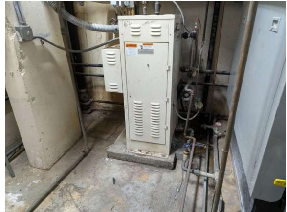
LKMC094e 1/27/2026 Steam generator for sterilizers SG-2 Boiler room
