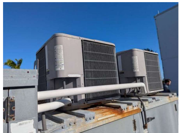
LKMC045e 1/27/2026 Ducted split system air-cooled condenser 1 North lower roof
