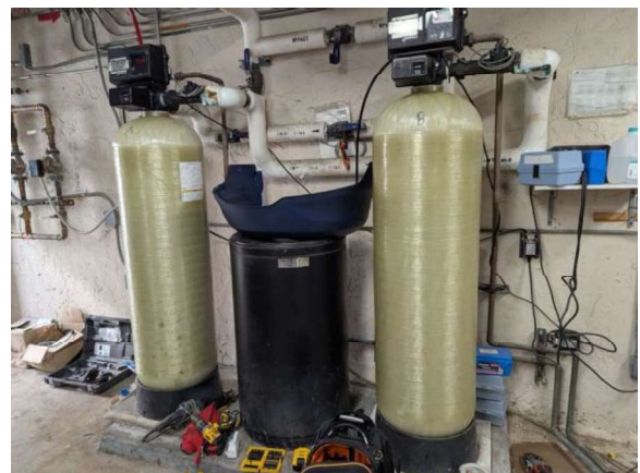
LKMC125e 1/27/2026 Water softener SOFT-1 First floor, southwest equipment room
