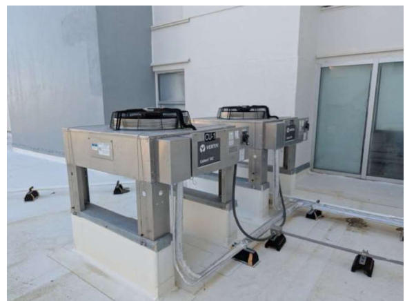
LKMC051e 1/27/2026 Ducted split system air-cooled condensers CU-1 and CU-2 North lower roof
