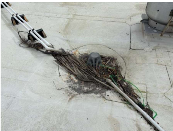
LKMC051a 1/27/2026 Roof drain with debris buildup Lower roof
