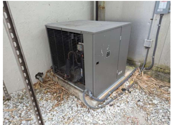
LKMC153e 1/27/2026 Refrigeration package for walk-in freezer North elevation
