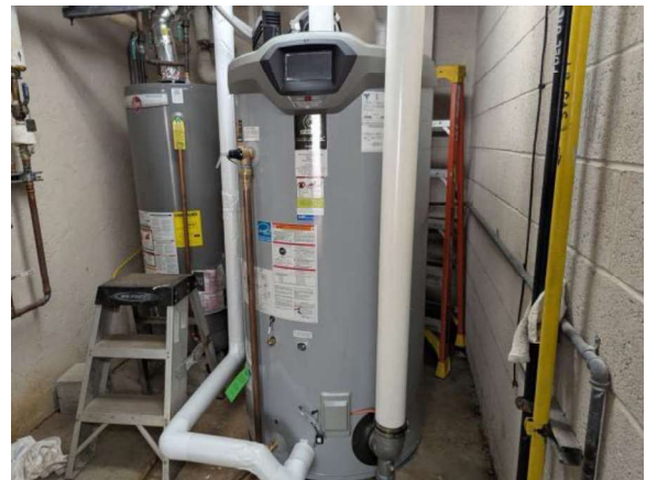
LKMC119e 1/27/2026 Commercial-grade, gas-fired domestic water heater First floor, southwest equipment room
