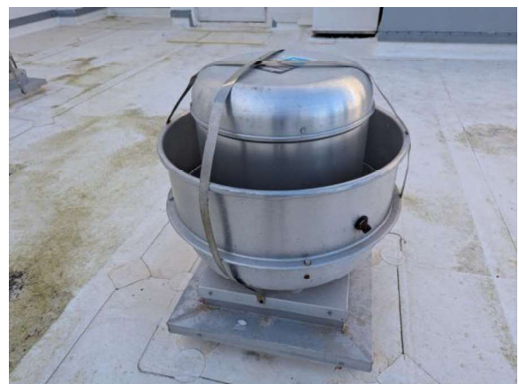
LKMC048e 1/27/2026 Centrifugal curb-mounted exhauster K-4 North lower roof
