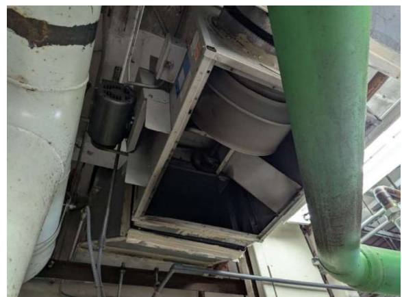
LKMC078e 1/27/2026 Inline centrifugal exhauster EF-25 Chiller room
