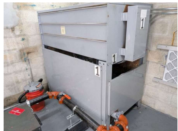
LKMC018e 1/27/2026 Hydraulic plant for passenger elevator ELEV-1 Elevator mechanical penthouse
