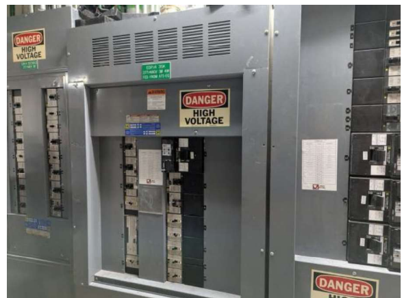
LKMC102e 1/27/2026 Electrical distribution load center EDP/A SECTION I Electrical room
