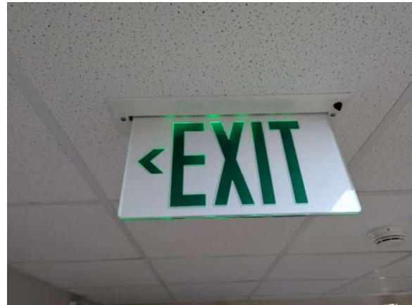
LKMC115e 1/27/2026 LED edge-lit blade emergency exit sign Suite 3-D
