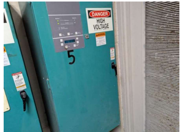
LKMC089e 1/27/2026 Automatic transfer switch ATS CH Emergency electrical room
