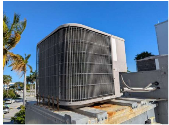
LKMC043e 1/27/2026 Ducted split system air-cooled condenser 2 North lower roof
