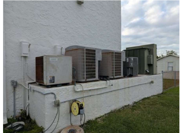
LKMC145e 1/27/2026 Ducted split system air-cooled condensers CND-4, CND-5, CND-6, and CND-7 East elevation
