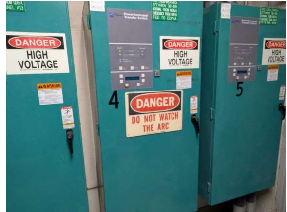
LKMC088e 1/27/2026 Automatic transfer switch ATS EQ Emergency electrical room
