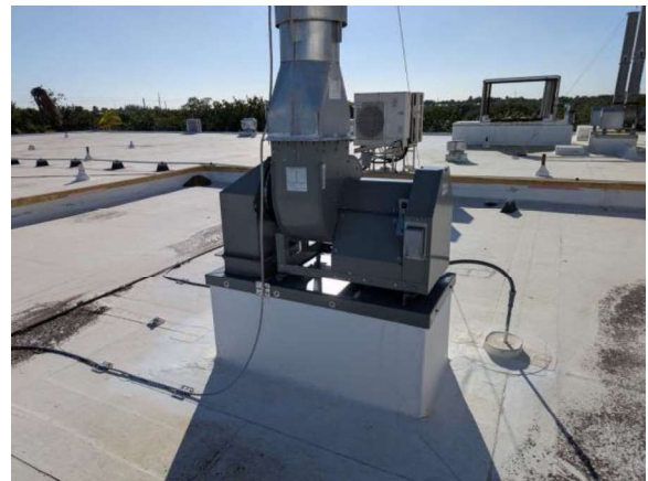
LKMC041e 1/27/2026 Utility set exhauster EF-1 NUC MED East lower roof
