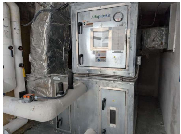
LKMC065e 1/27/2026 Indoor air handler AHU-6 First floor, southeast mechanical room
