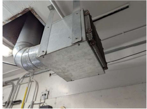
LKMC064e 1/27/2026 Propeller-style ventilation fan SF-1 Compressor room
