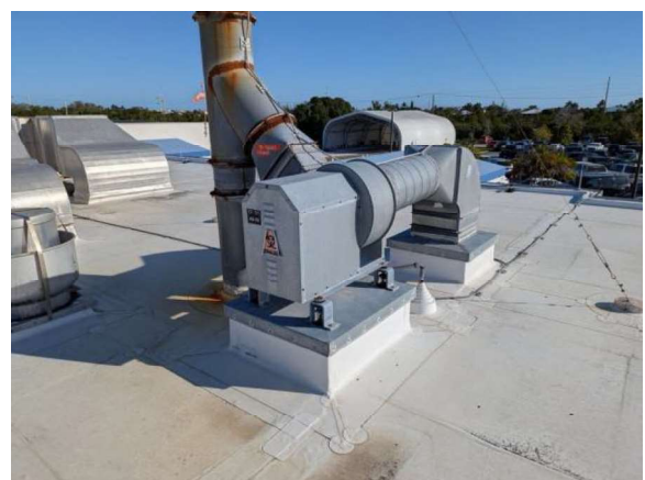
LKMC030e 1/27/2026 Utility set exhauster EF-3A East lower roof
