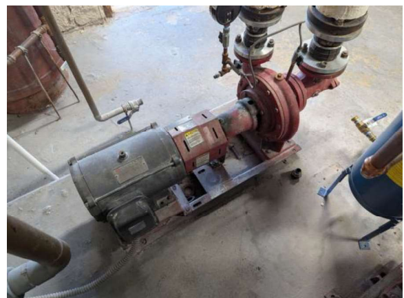
LKMC099e 1/27/2026 Heating water pump HWP-1 Boiler room
