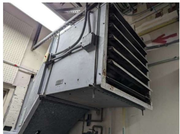
LKMC095e 1/27/2026 Propeller-style ventilation fan SF-3 Boiler room
