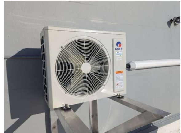
LKMC016e 1/27/2026 Air-cooled condenser for ductless split system DDXS-D Upper roof
