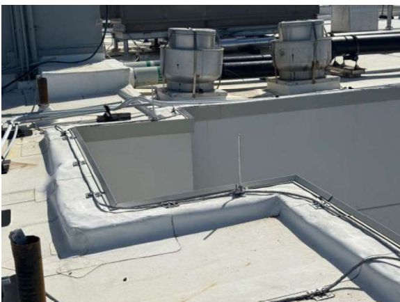
LKMC003a 1/27/2026 Single-ply white membrane parapet detail and lightning protection Upper roof
