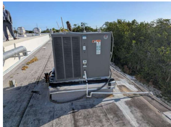
LKMC020e 1/27/2026 Package air conditioning unit RTU-2 East lower roof
