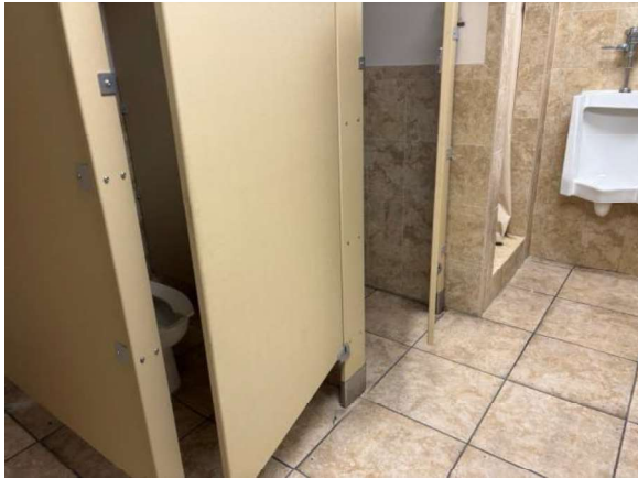
LKMC061a 1/27/2026 Tiled surfaces, nonaccessible shower, and nonaccessible water closets First floor, men's locker room
