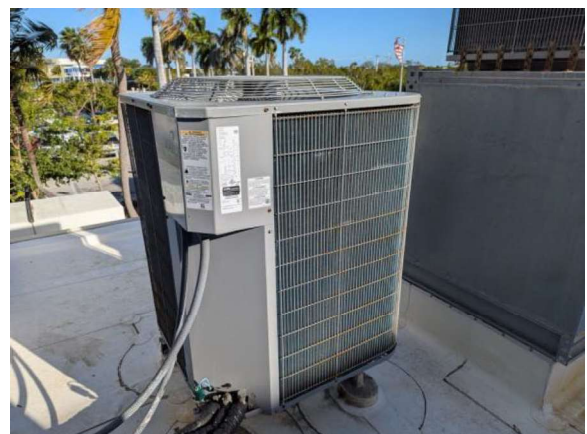
LKMC042e 1/27/2026 Ducted split system air-cooled condenser CNDR-9 North lower roof
